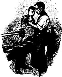
Fig. 7.—Winding an Armature.
